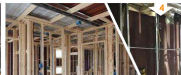
4 Framing, Electrical, & Plumbing
